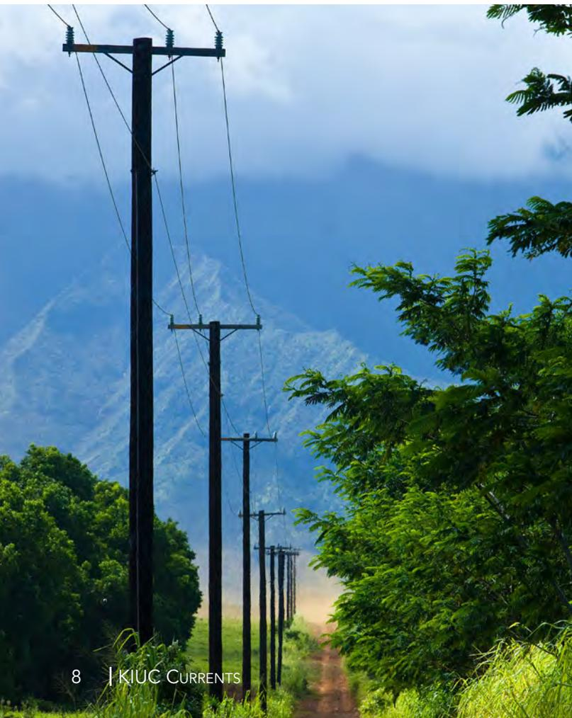
**Utility Pole** — Partially buried to support all of the equipment. It usually is about 40 feet long and typically made from logs.
