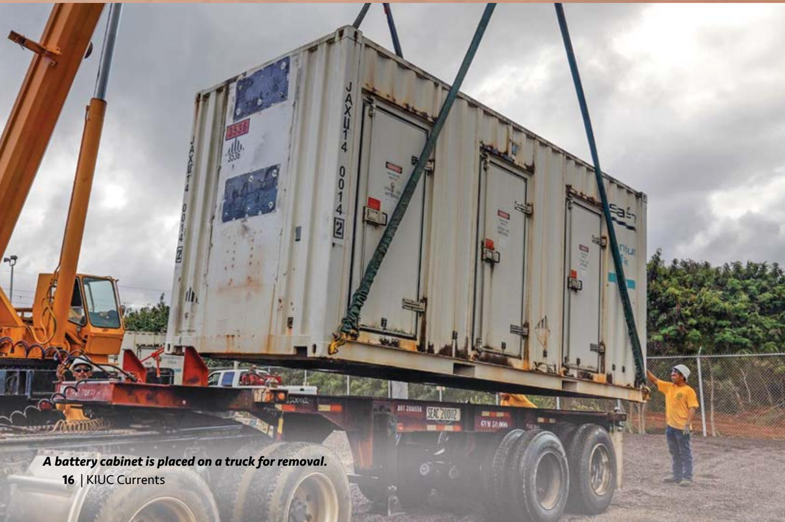
**A battery cabinet is placed on a truck for removal.**
