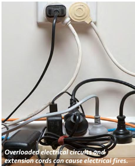
Overloaded electrical circuits and extension cords can cause electrical fires.
