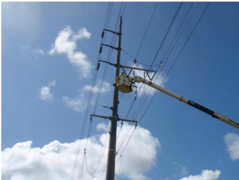
9) Structure 2 – Installed lower transmission arm and assemblies.
