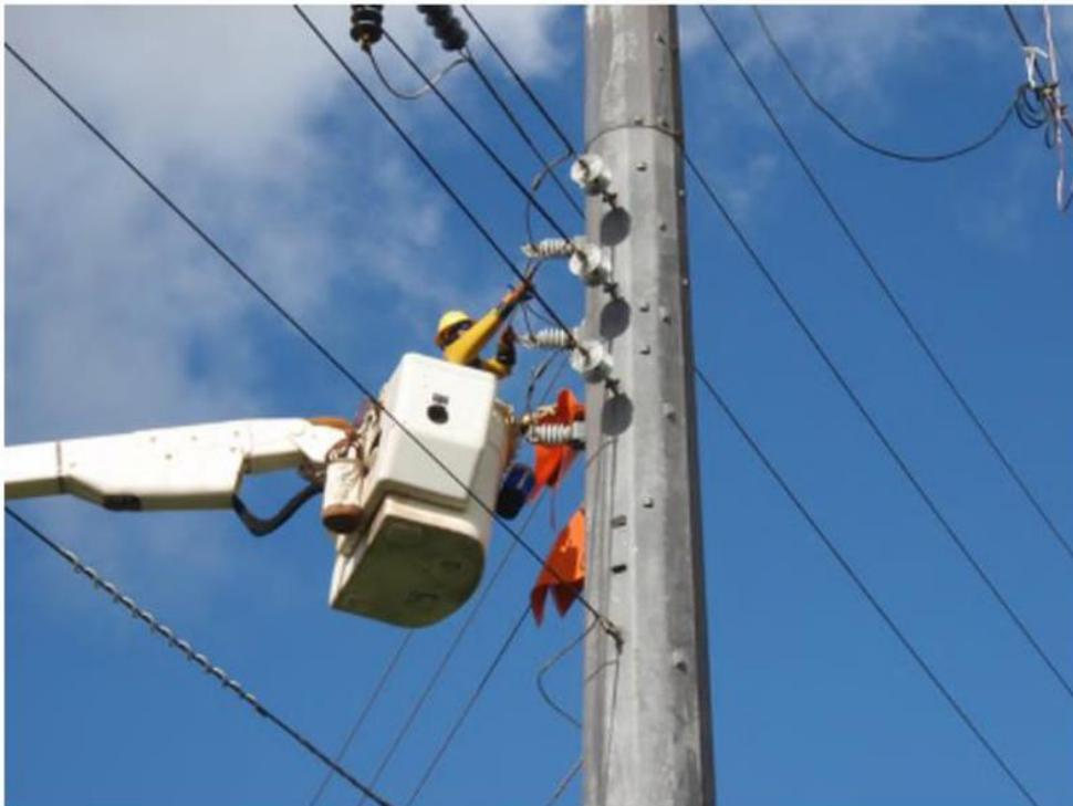
4) Structure 1 – KIUC crew cutting jumpers on structure 1 to de-energize the line.<sup>6</sup>
