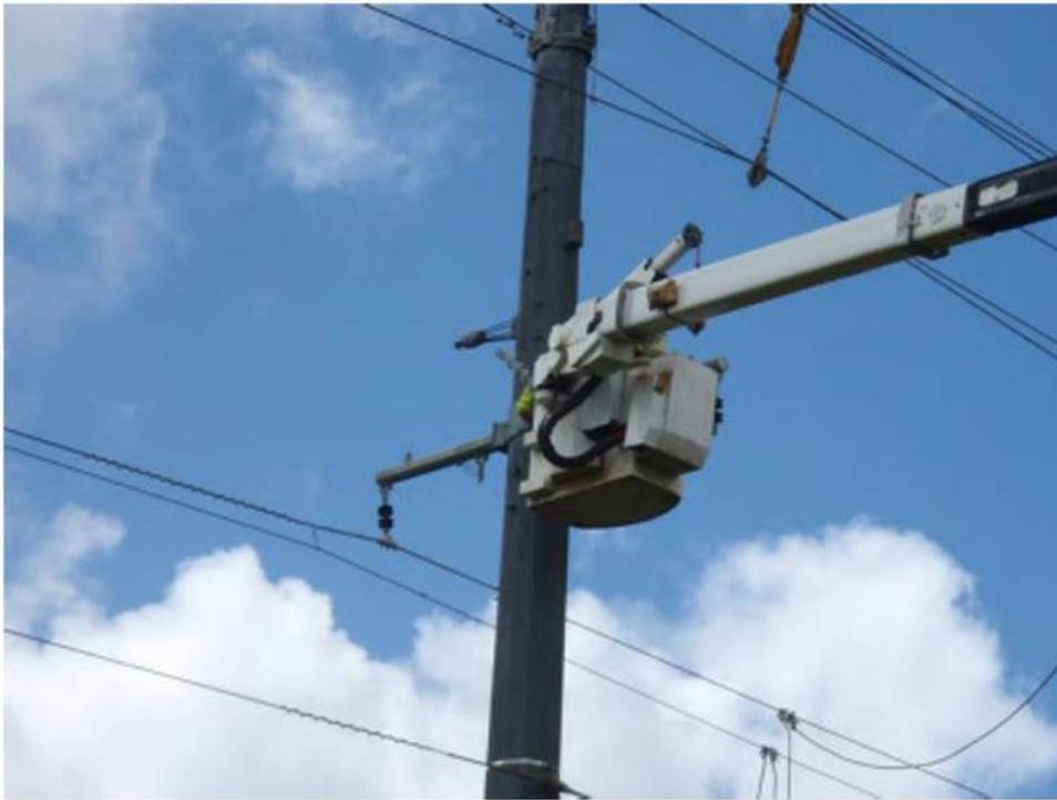
6) Structure 2 – Welder finished distribution welding. Distribution arms installed.<sup>6</sup>
