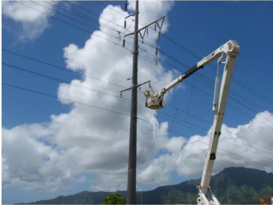
7) Structure 2 – Installing conductor in rollers (other than neutral.)
