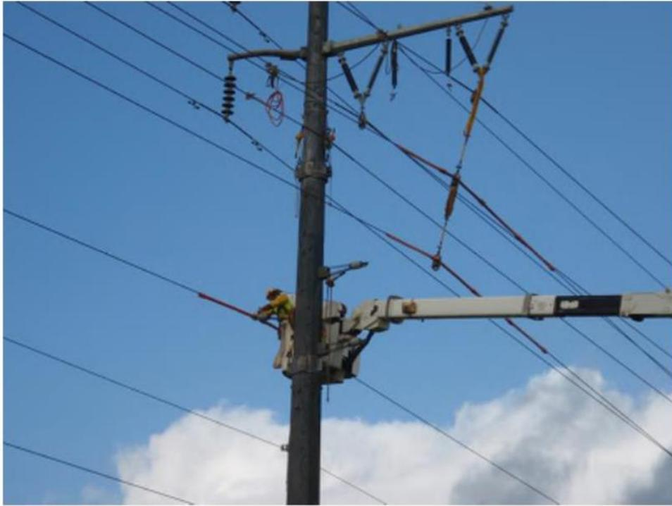
5) Structure 2 – Spreading and covering distribution so welder can finish on weld.<sup>7</sup>
