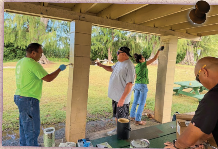
KIUC staff spent a community service day refreshing the Niumalu Park Pavilion.
