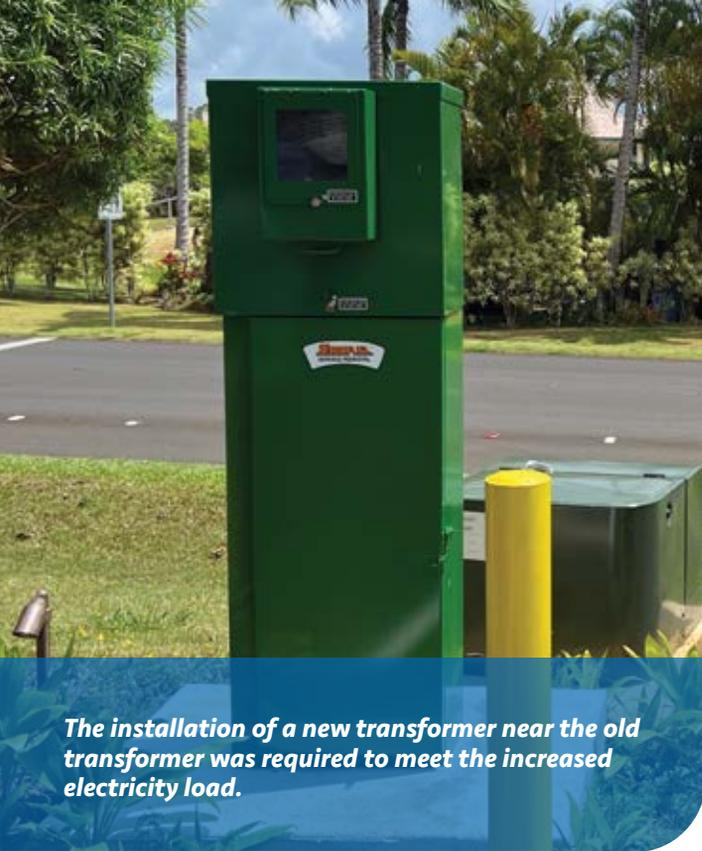
*The installation of a new transformer near the old transformer was required to meet the increased electricity load.*
