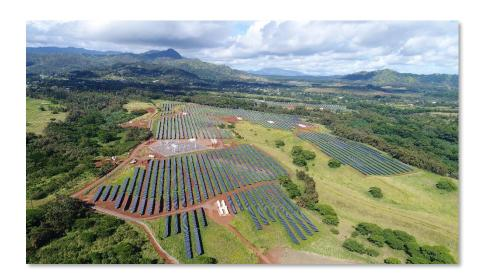
The AES Lāwa'i solar-plus-storage facility can provide up to 20 megawatts of direct-to-grid power during the day, along with five hours or 100 megawatt hours of electricity for use after sunset. *Photo credit: AES*
