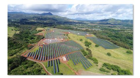
The AES Lāwa'i solar-plus-storage facility can provide up to 20 megawatts of direct-to-grid power during the day, along with five hours or 100 megawatt hours of electricity for use after sunset.
